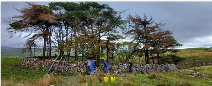
In September 2020, CNCC volunteers spent a wet day rebuilding sections of drystone wall around Alum Pot which protects visitors and livestock. A 5m section was rebuilt completely and another six sections were repaired where the top had fallen.
